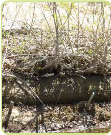
Bioengineering techniques, for example wattles and willow cuttings, are used to repair stream banks.
