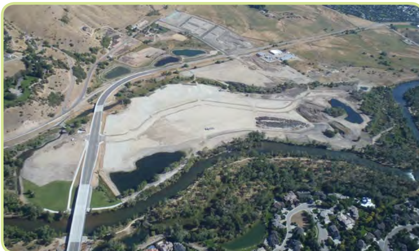
| Marianne Williams Park under construction. |
