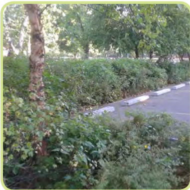
The parking lot at Municipal Park drains to a vegetated swale, an example of green infrastructure.
