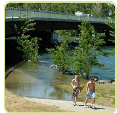
Parts of the Greenbelt path flood during high water caused by spring runoff.
