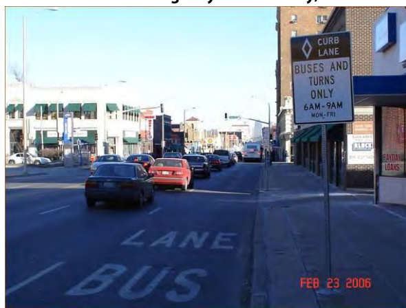
Curbside Running Way – Kansas City, Missouri
