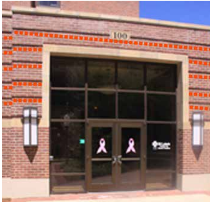
Recessed brick creates horizontal bands around the perimeter at St. Luke's Boise facility.
