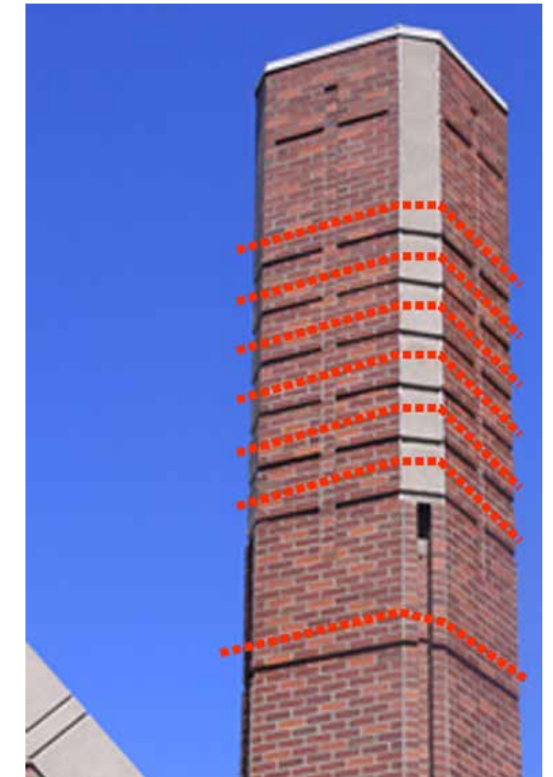
The arrangement of brick through relief and banding creates symbolism at St. Luke's Boise facility.
