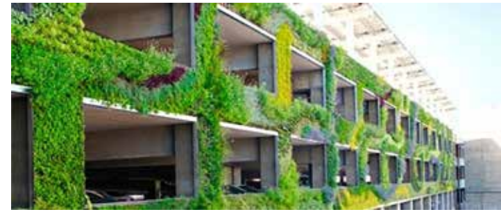
Example of "green wall" treatment applied to the facade of a garage.
