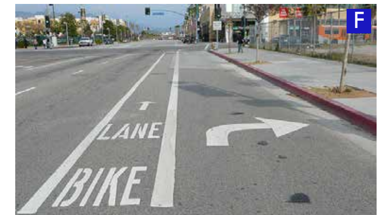
Example of a through bike lane.
