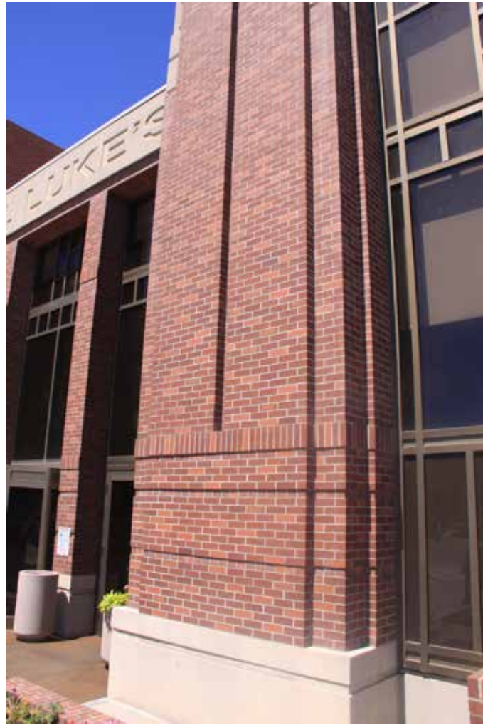
A column at the St. Luke's Boise facility that has vertical relief and horizontal relief to help identify the main entry.
