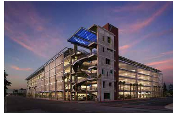
Dissolution of typical garage features like stair and elevator cores to provide visual interest and activation.
