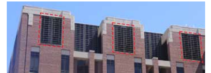
Mechanical grilles are used and arranged in the same fashion as glazing to break up and divide exterior walls.
