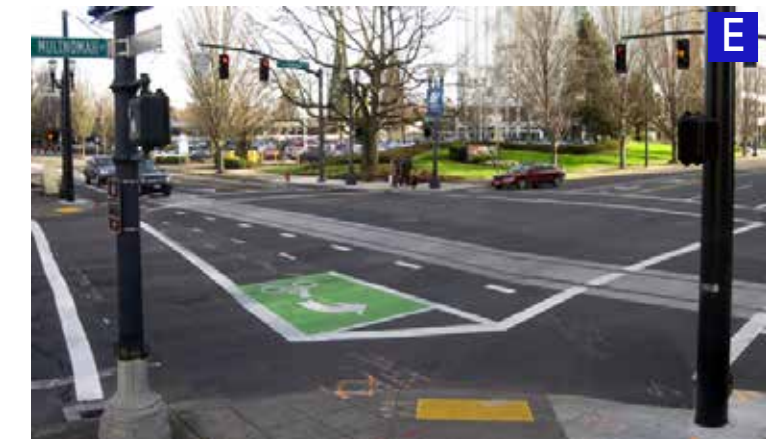
Example of a two-stage turn queue box.
