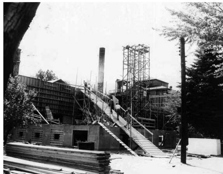
Constructing St. Luke's "Million Dollar Wing," 1951.
