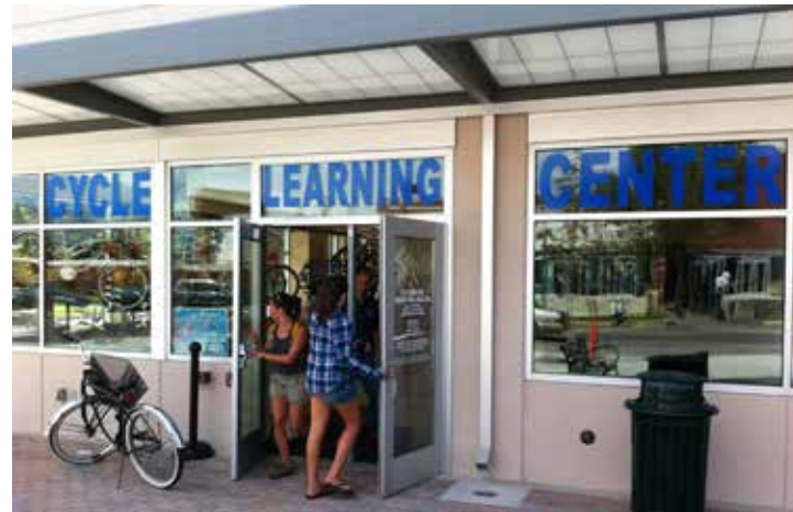
Existing example of ground floor developed retail within a garage at Boise State University.
