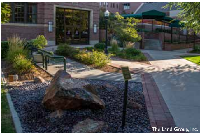
The Land Group, Inc. Permeable pavers and bio-retention designed into pedestrian circulation.
