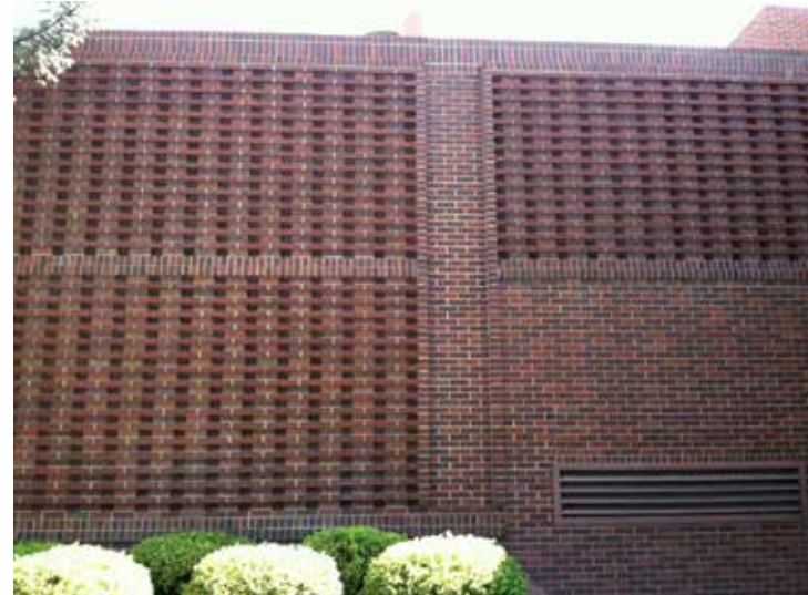
Brick used as a screen for mechanical equipment at St. Luke's Boise Medical Center creates an ornamental pattern on the building exterior.
