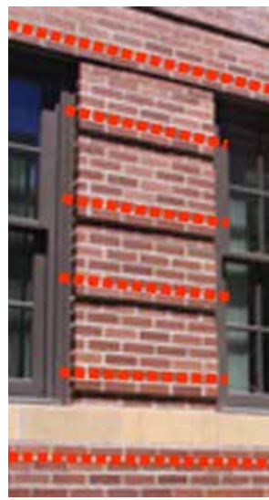
Banding in the brick aligns with adjacent building elements, tying together separate parts of the building.
