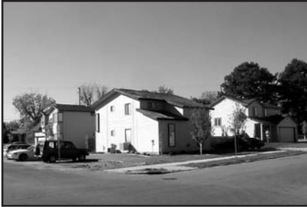
These three homes at the corner of Lincoln Avenue and Rossi Street were built on property zoned for apartments.
