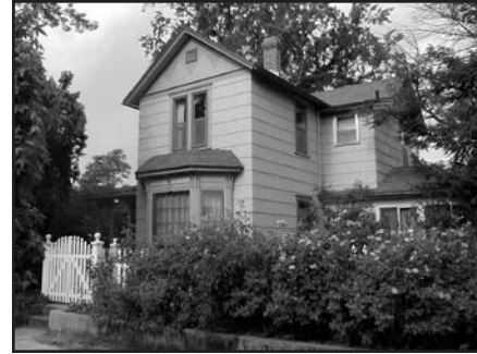
This newer duplex at left on Denver Avenue was built in a C-2D zone. Design review helped it blend into the neighborhood of older homes like the one above, which is located across the street.
