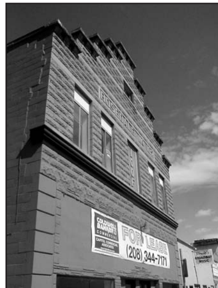
The old South Boise business area might benefit from streetscape improvements like those downtown on Eighth Street.
