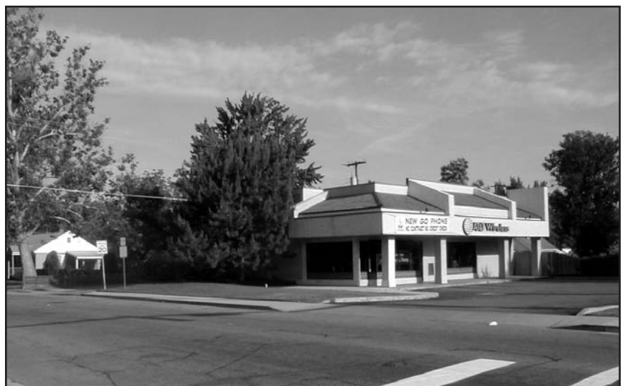
The AT&T Wireless building on Broadway backs up to the alley, forming a barrier between its parking lot and the residence behind it on Highland Street.
