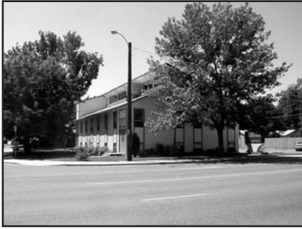
The University Baptist Church, seen from Beacon Street.
