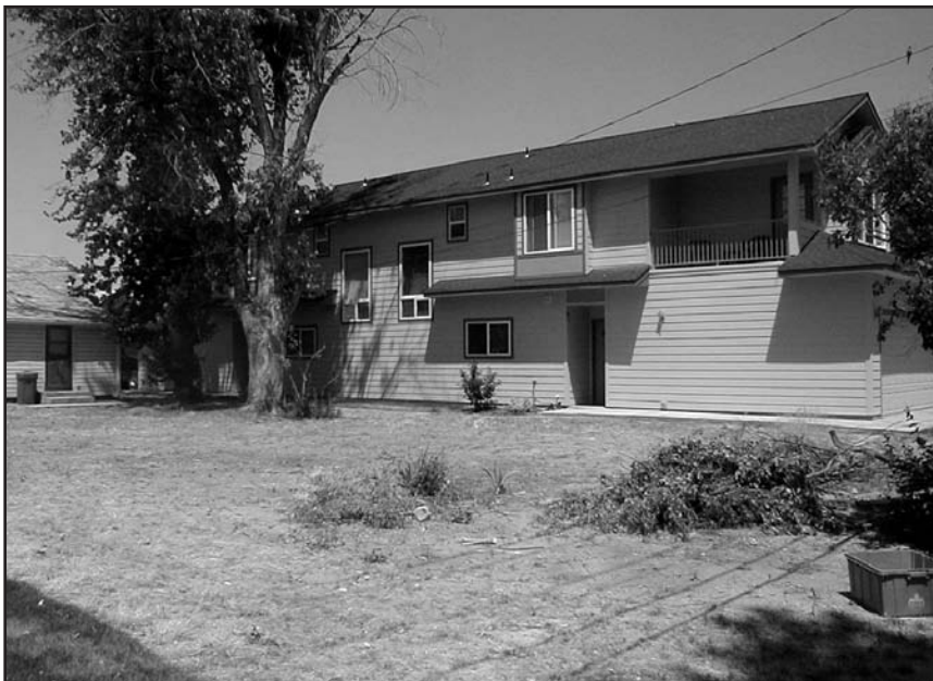
The balcony on the rear unit of this 20 by 90-foot duplex on Manitou Avenue looks directly into the backyard of the small historic house next door at left.
