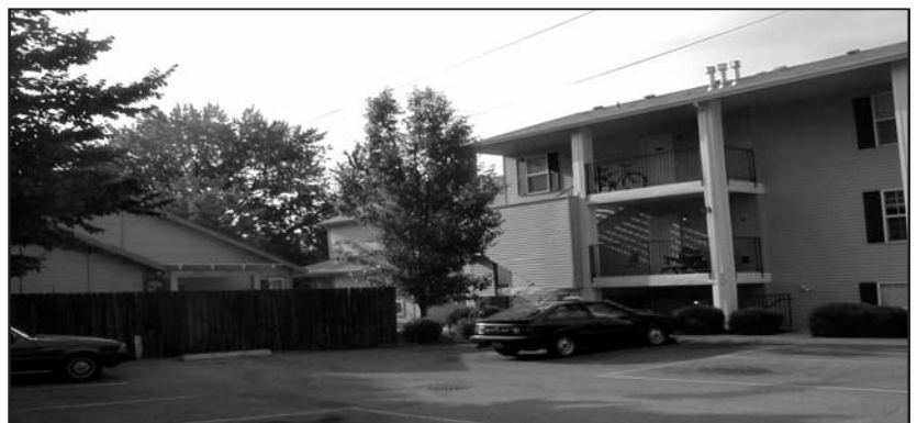
This 2.5 story quad triplex on Euclid Avenue has porches and living room windows that look down into the back yards of neighbors on both sides.
