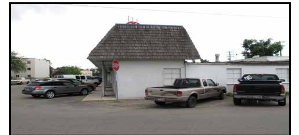
Figure 25 - Existing on-street parking for businesses
