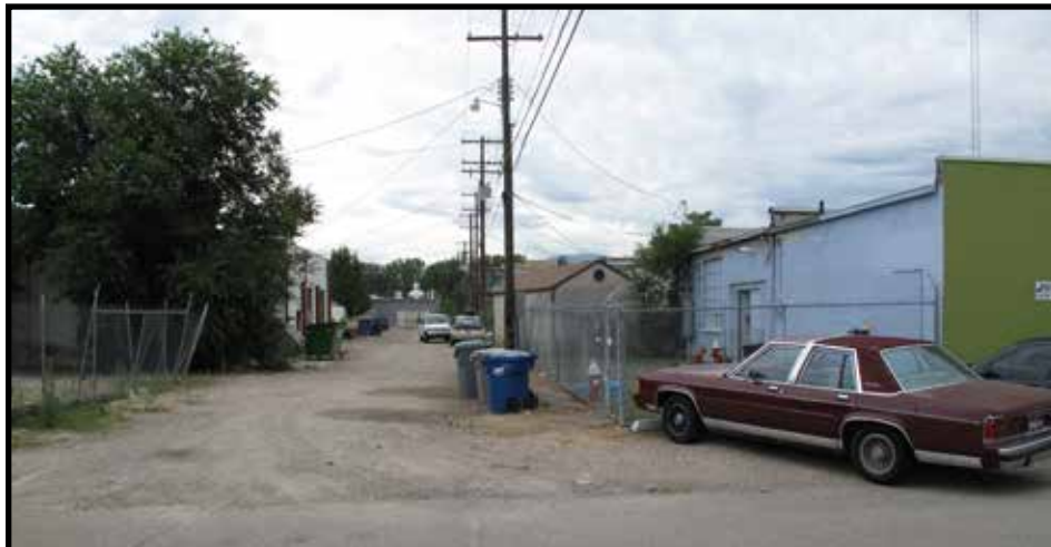
Figure 27 - Power lines that could be undergrounded when redevelopment occurs.
