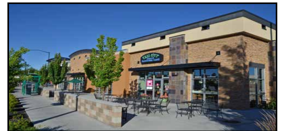
Figure 4 New construction in the area
