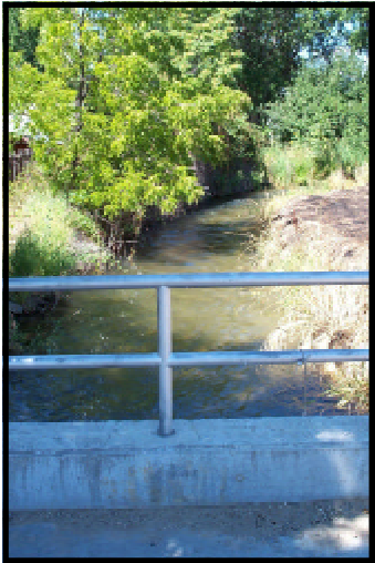
Canal Bridge near Ustick Road
