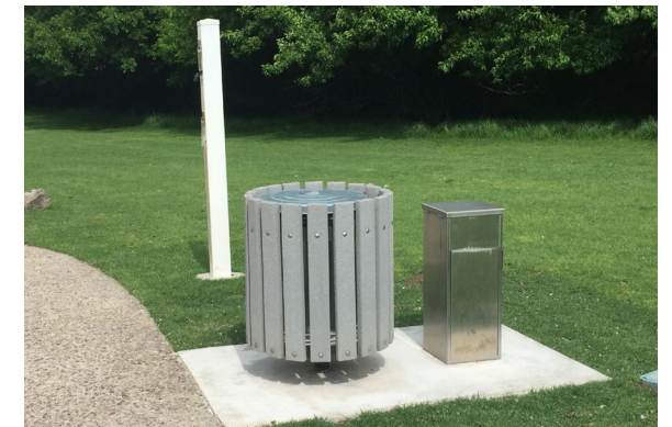
○ ■ SITE PHOTO #5 REMOVE CONCRETE AT TRASH RECEPTACLE, TRASH RECEPTACLE & DOG WASTE STATION
