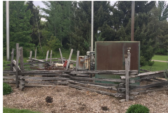
○ ■ SITE PHOTO #8 REMOVE WOODEN FENCE
