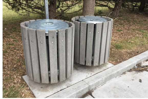
○ ■ SITE PHOTO #2 REMOVE CONCRETE & TRASH RECEPTACLE
