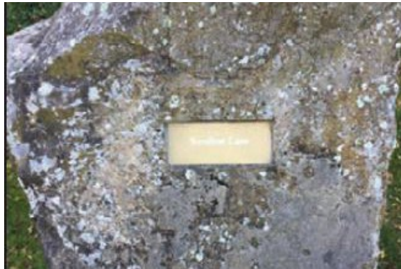
○ SITE PHOTO #7 REMOVE 5"X12" BOULDER PANELS (EXAMPLE)
