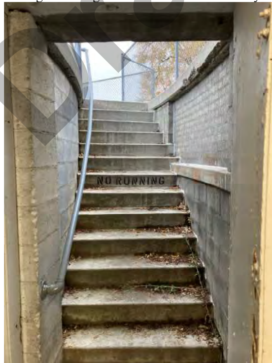
Stair from men's restroom up to pool deck.
