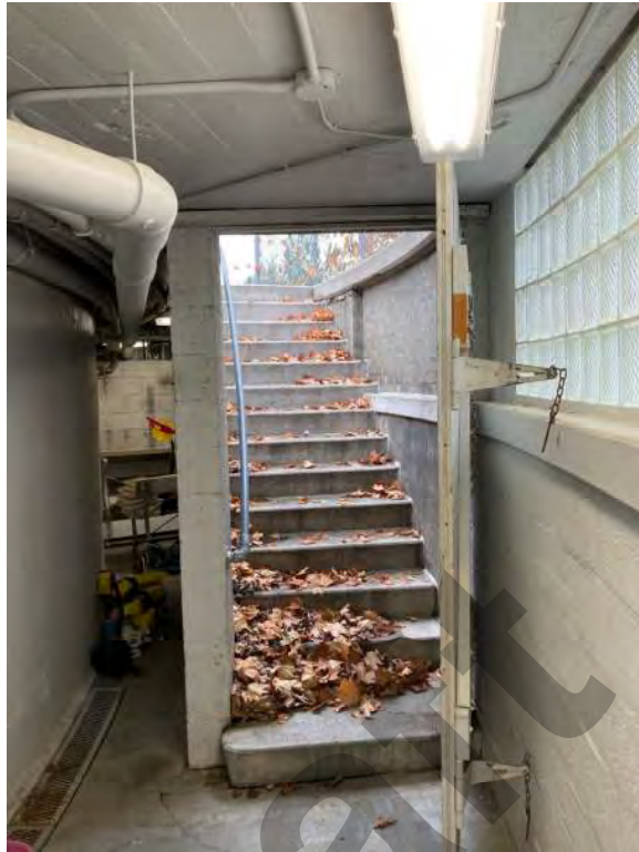
Stair from men's changing room to pool deck.
