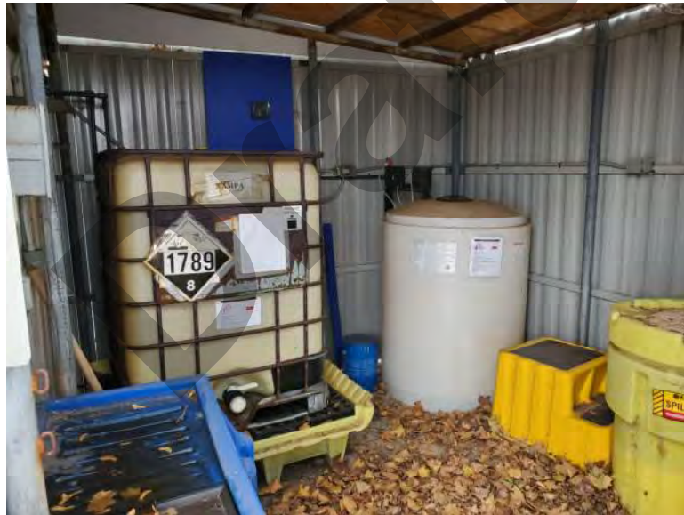
Another image of the pool equipment storage shed at far west side of facility.
