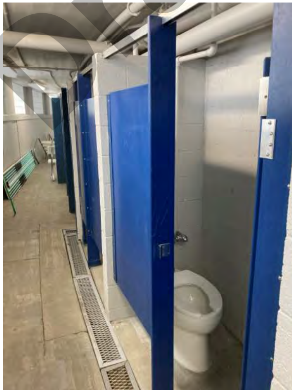
Toilet partitions and fixture.
