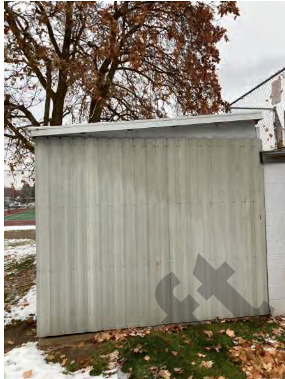
Pool equipment storage shed at far west side of facility.
