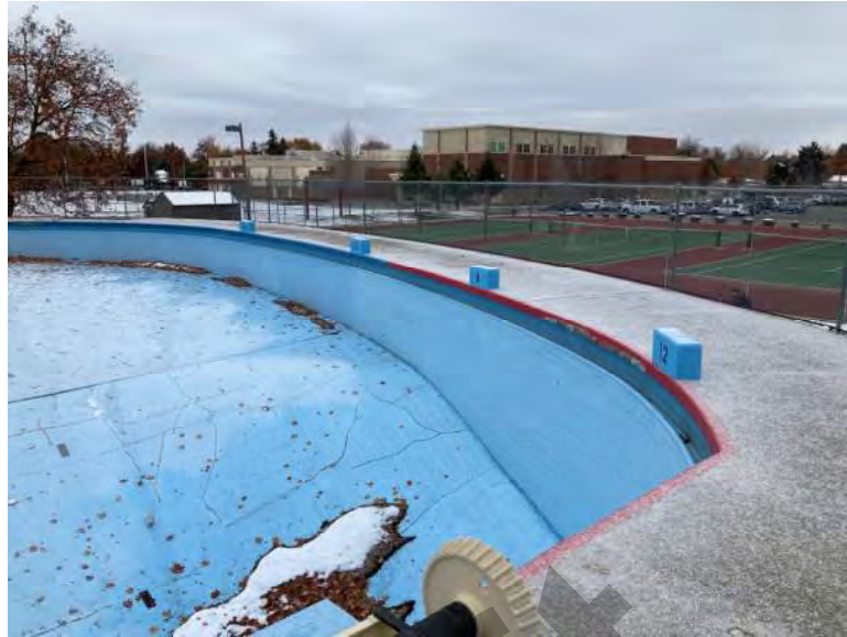
Pool and pool deck.
