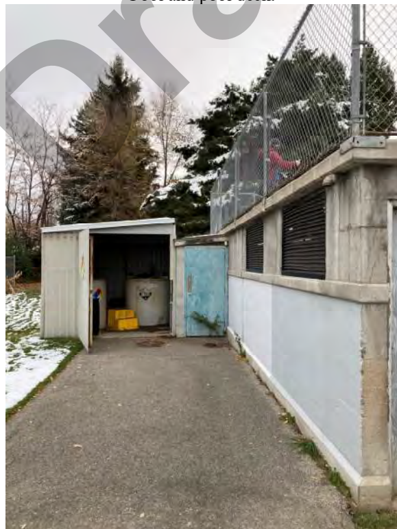
Storage shed at far west side of facility.
