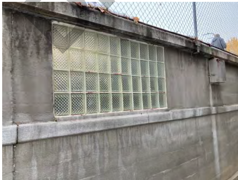
Glass block opening at exterior wall.
