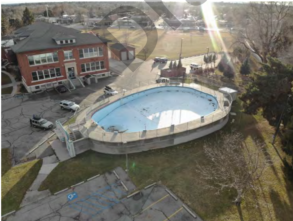
Axon view, looking southwest, of pool deck at the Lowell pool. Image taken by Cushing Terrell via drone photography.
