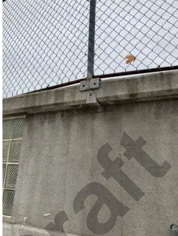
Fence post attachment to concrete edge.
