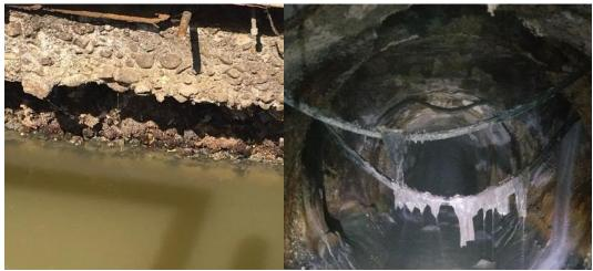
Figure 1 - Examples of degrading water renewal infrastructure. Left degrading concrete at the Lander Street Water Renewal Facility. Right degrading pipe in the collection system
